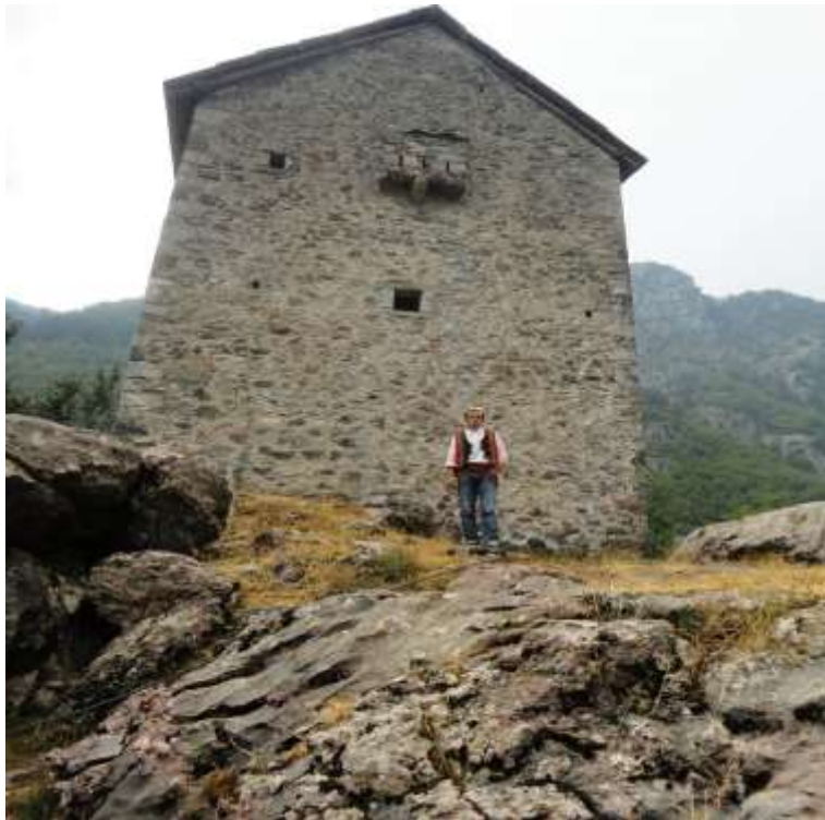
Fig. 3. Tower of Detention - Theth (Photo by Q. Kastrati, 2014.)
